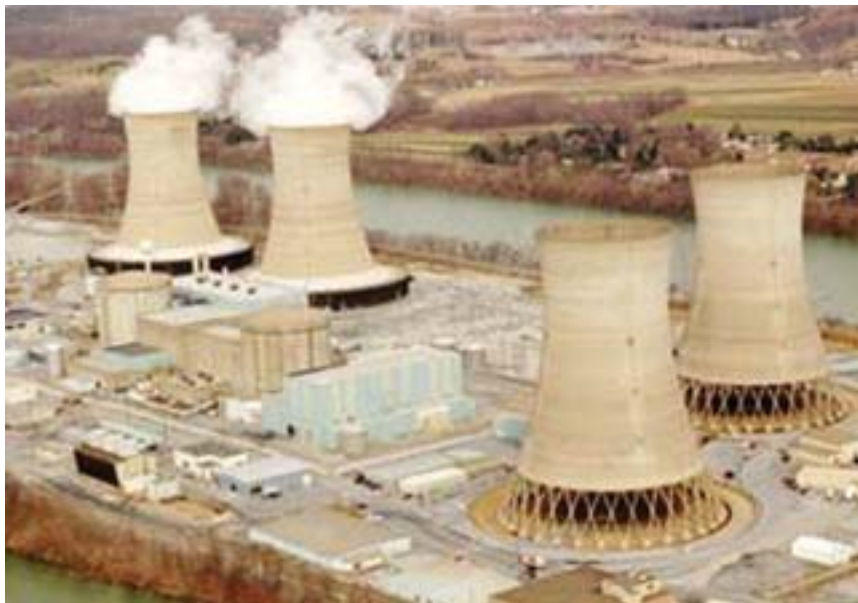
Nuclear Power Station
