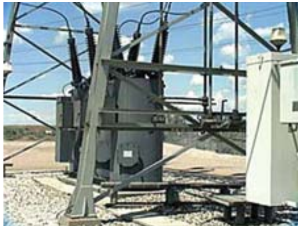
Oil circuit breaker
